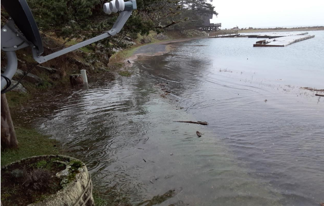
January flooding under office and lagoon drive
