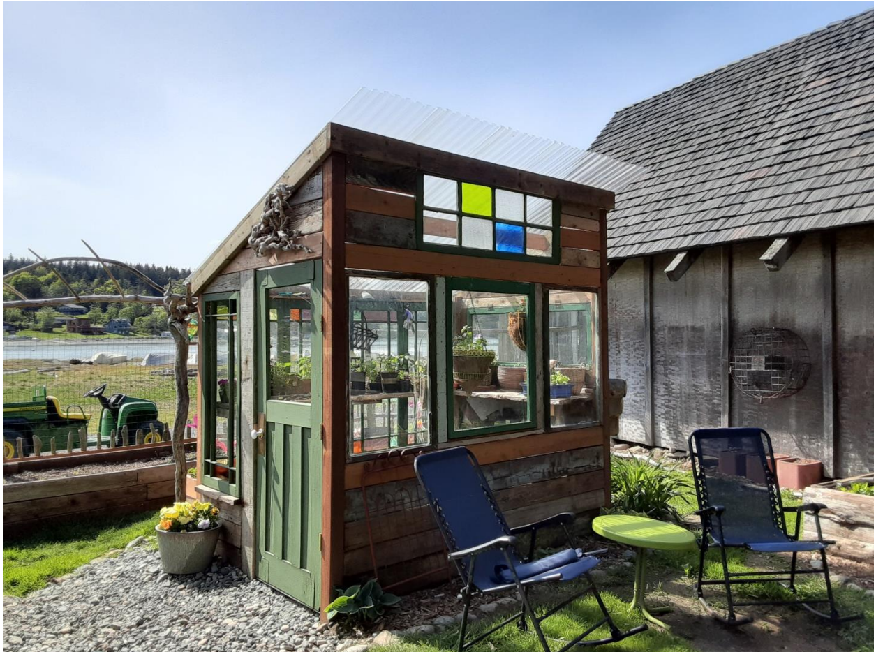
Back of the greenhouse. More donated windows and door...with a little color added
