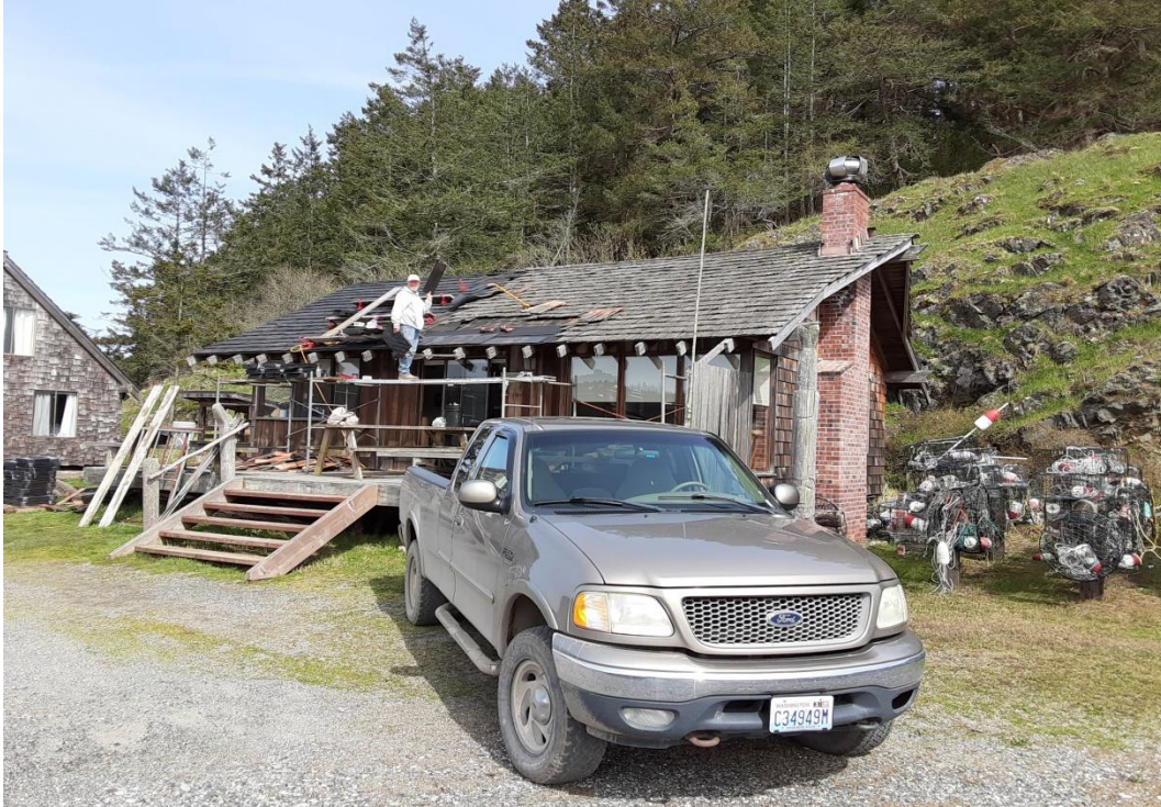
Maintenance Man at work again. Work in progress.
