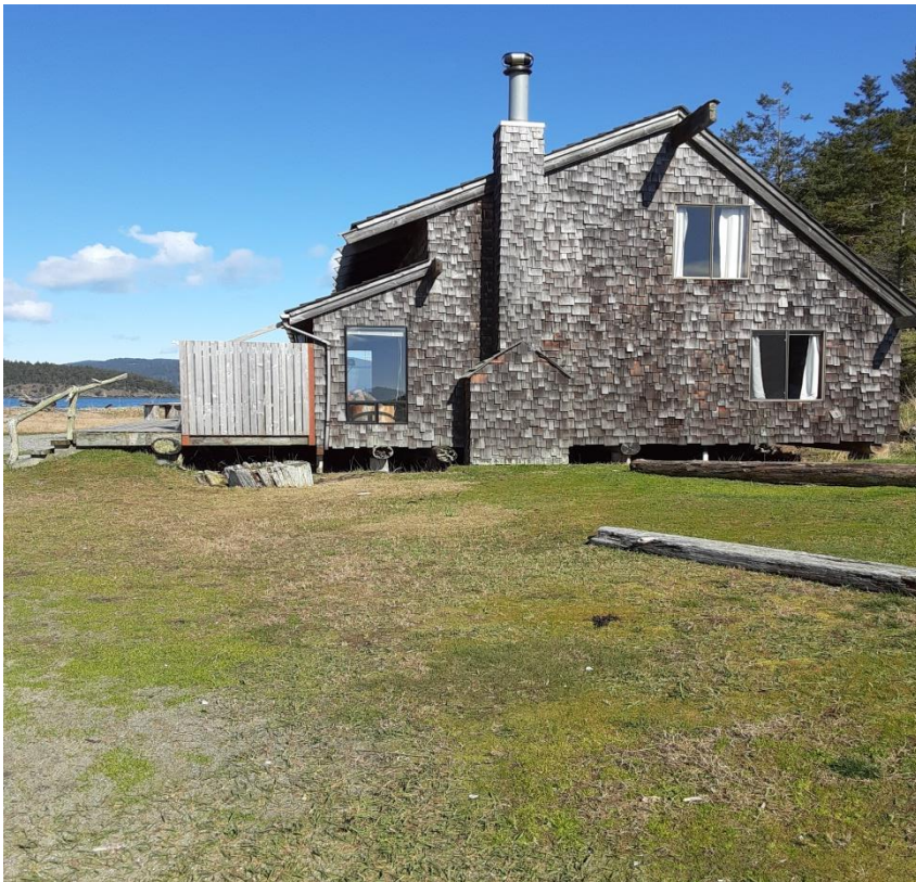
After clean-up. Large logs were removed with backhoe a few weeks ago
