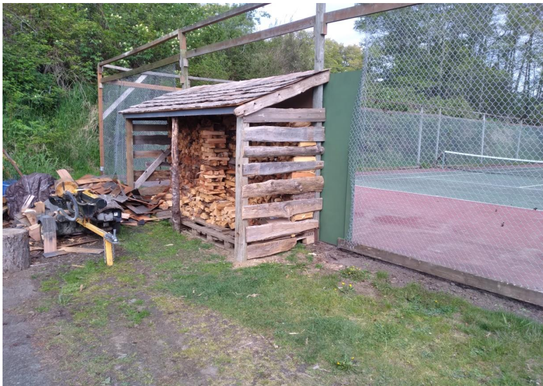
New firewood storage shed and support for backboard
